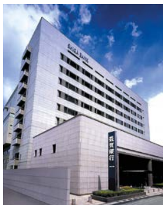
Shiga Bank Head Office
